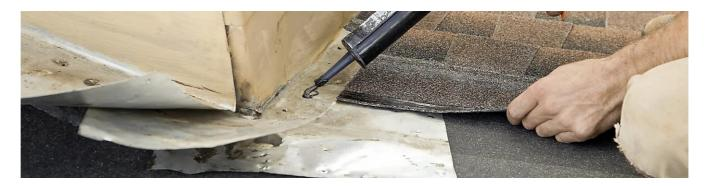
Shell Tixophalte is a filler, joint sealer and adhesive. This highly versatile bituminous compound is a high performing and versatile sealant solution for industry professionals and DIY enthusiasts alike.
